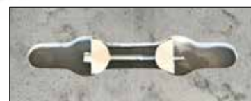
Use Compact Laminite Jig to rout cut outs for toggle bolts
